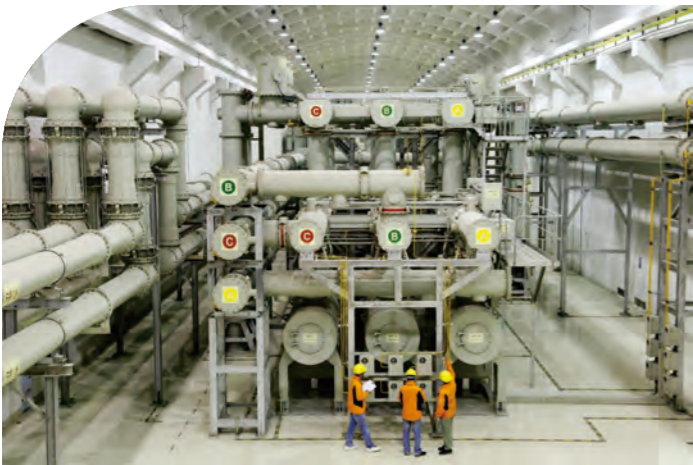
四川省雅砻江锦屏二级水电站机电设备安装工程监理(含GIS设备制造及安装监理) Mechanical and Electrical Equipment Installation Engineering Supervision of Yalong River Jinping II Hydropower Station, Sichuan (including GIS Equipment Manufacturing and Installation Supervision) 变电站电压等级500kV，线路电压等级500kV Substation voltage level: 500kV, line voltage level: 500kV
